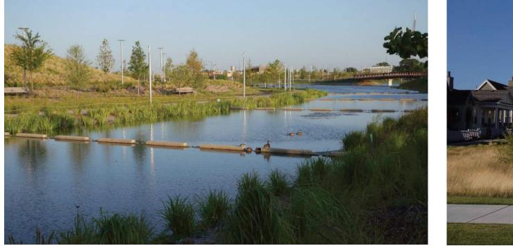
Step pools of a stormwater chain during a high-water runoff event
